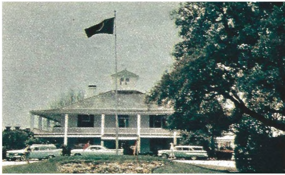
A landmark is the old manor house.
